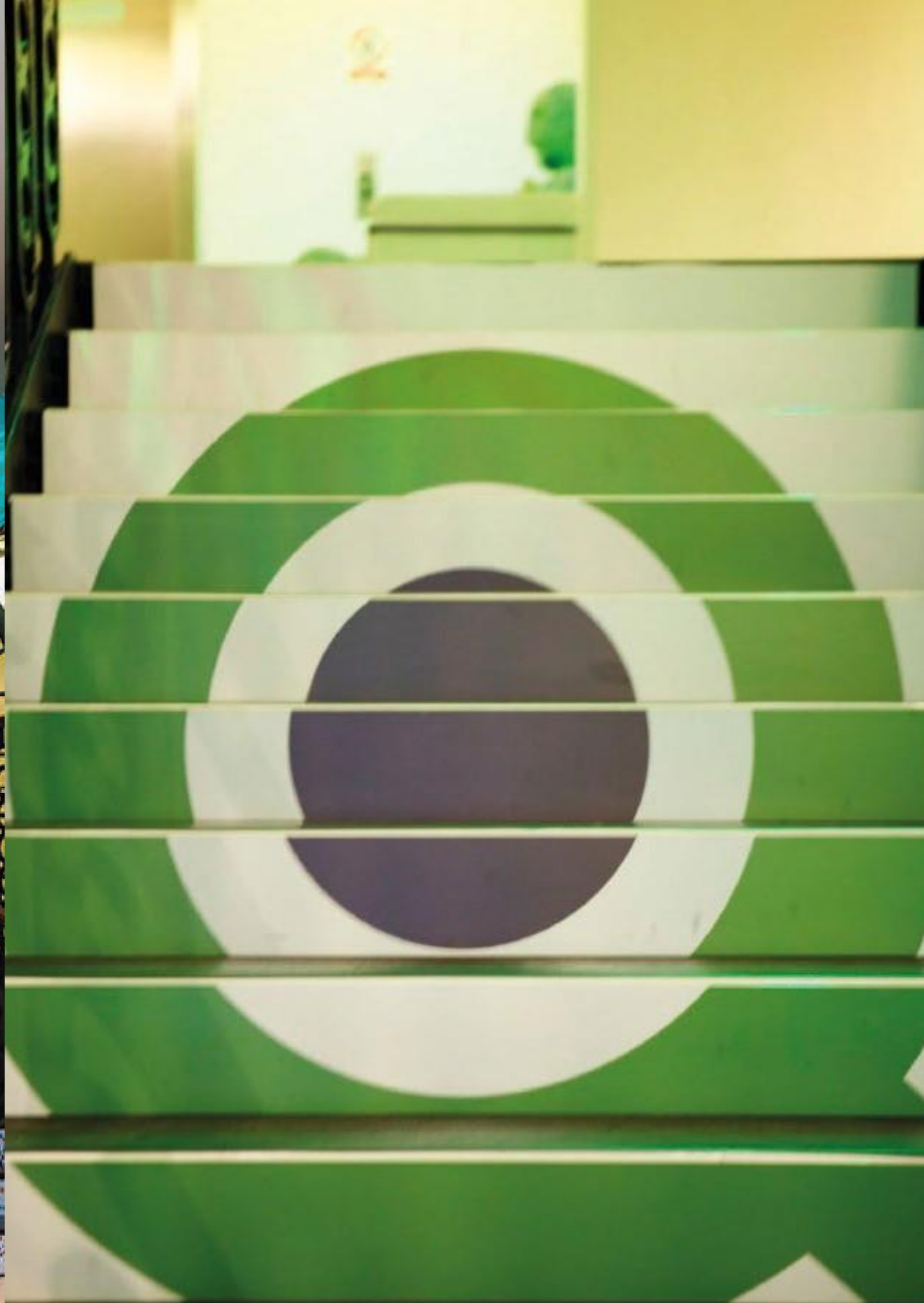
Stairs C1 & C2
